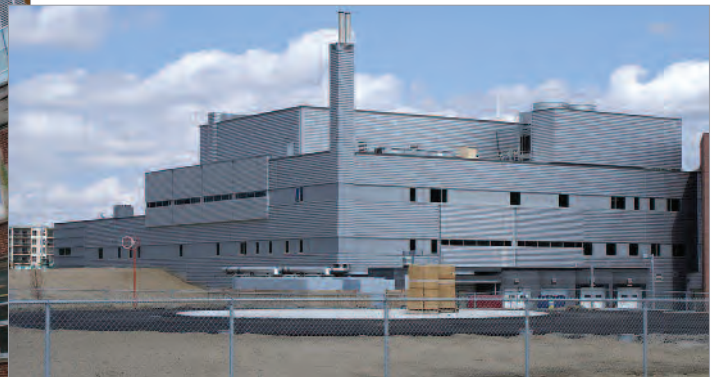
WOODSTOCK HOSPITAL Aluminum Panel System, Prefinished Metal Cladding, Insulated Metal Panel, Steel Roof Deck
