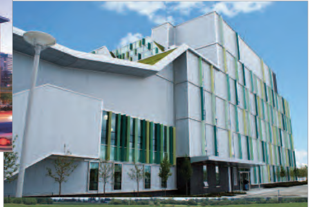
CENTRE FOR CONSTRUCTION EXCELLENCE, ALGONQUIN COLLEGE, OTTAWA Insulated Metal Panel, Composite Metal Panel System
