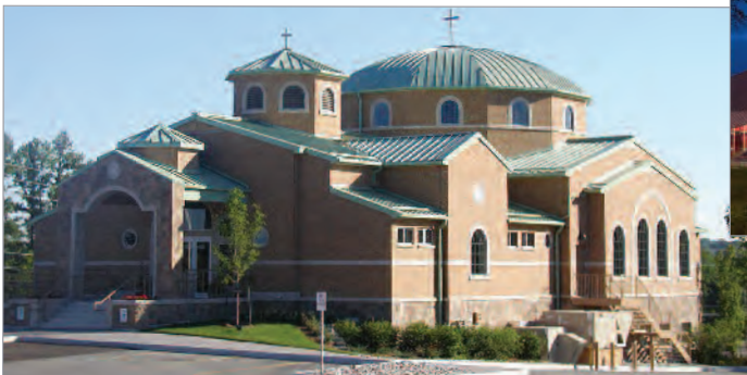
ST. DIMITAR CHURCH, BRAMPTON Prefinished Metal Roofing and Cladding
