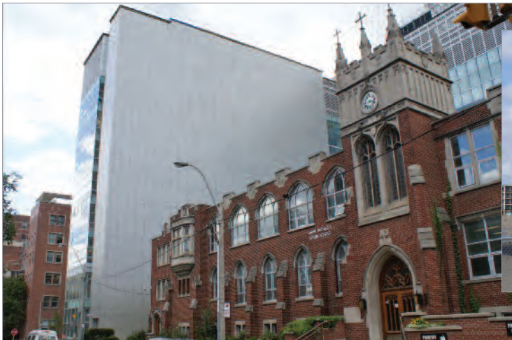
LI KA SHING KNOWLEDGE INSTITUTE, ST. MICHAEL'S HOSPITAL Aluminum Panel System, Prefinished Metal Cladding
