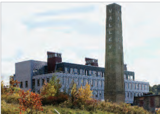
EVERGREEN BRICK WORKS, TORONTO Fibre Cement Cladding, Prefinished Metal Cladding, Composite Metal Panel System
