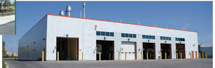
MISSISSAUGA TRANSIT BUS GARAGE Insulated Metal Panel, Prefinished Metal Cladding, Explosion Relief Panel
