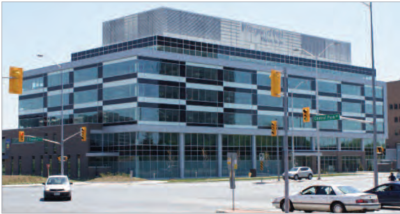
REGION OF PEEL - JOINT USE FACILITY, BRAMPTON Aluminum Panel System, Prefinished Metal Cladding
