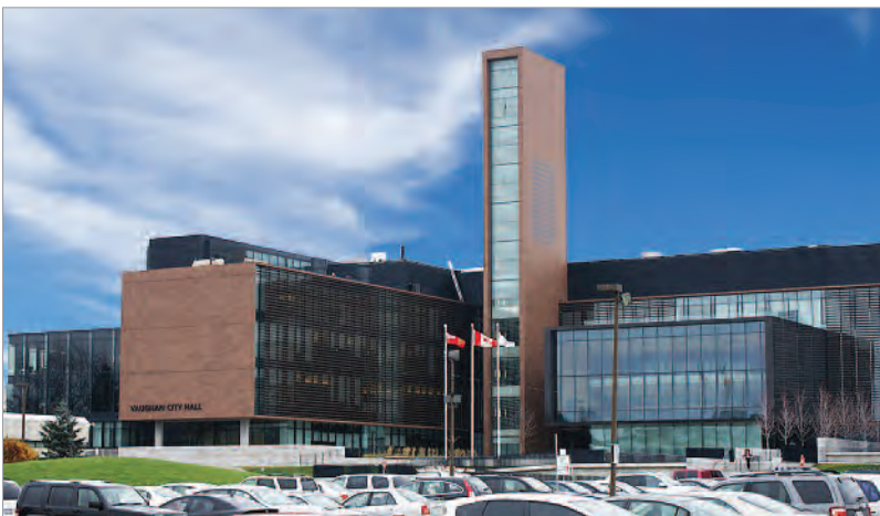
VAUGHAN CITY CENTRE Terra Cotta Panel, Aluminum Panel System
