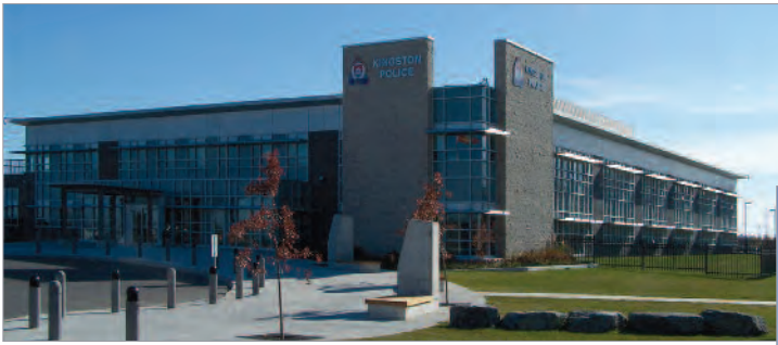
KINGSTON POLICE, KINGSTON Composite Metal Panel System, Prefinished Metal Cladding
