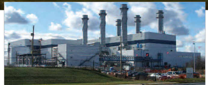
SITHE GLOBAL POWER STATION - BRAMPTON Prefinished Metal Cladding
