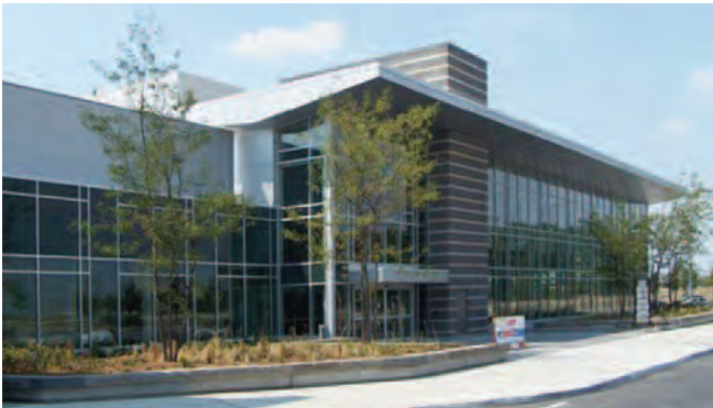
HERSHEY CENTRE, MISSISSAUGA Insulated Metal Panel, Composite Metal Panel System, Kalwall Translucent Panel System
