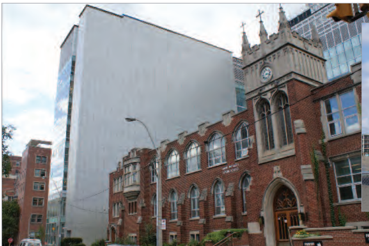
LI KA SHING KNOWLEDGE INSTITUTE, ST. MICHAEL'S HOSPITAL Aluminum Panel System, Prefinished Metal Cladding
