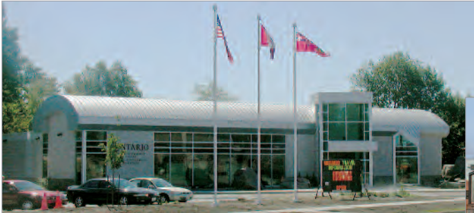
BLUE WATER BRIDGE, SARNIA Composite Panel System, Prefinished Metal Roofing and Cladding
