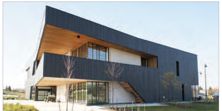
SKI CHALET, CHINGUACOUSY PARK, BRAMPTON Zinc Cladding, Prefinished Metal Cladding, Aluminum Panel System
