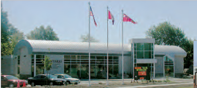
BLUE WATER BRIDGE, SARNIA Composite Panel System, Prefinished Metal Roofing and Cladding
